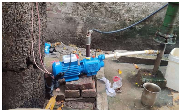
Figure 3: Suction Motor and Hand pump connected to a borehole
